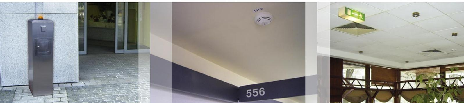
During a fire alarm, a fire brigade key deposition facilitates perpetual easy access and passage to all rooms protected with fire detectors and/or automatic extinguishing systems.
